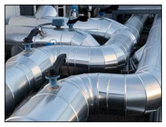
Aeroflex USA does not recommend specific protective jacketing systems. However, the specified and installed system should be sized correctly so it does not compress the insulation. See "Cladding | Jacketing" schedule under Technical Resources for Aerocel pipe insulation OD's.
